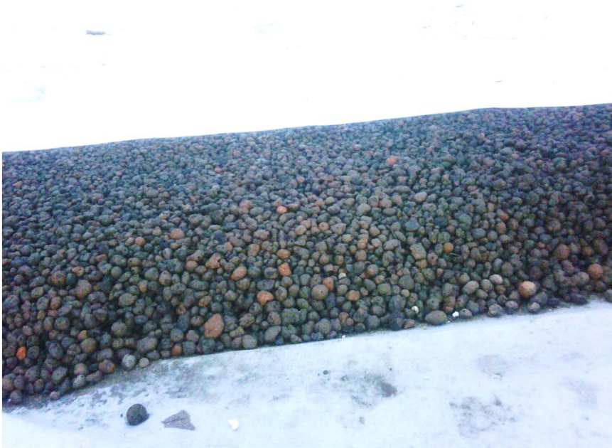
Granular drainage layer
